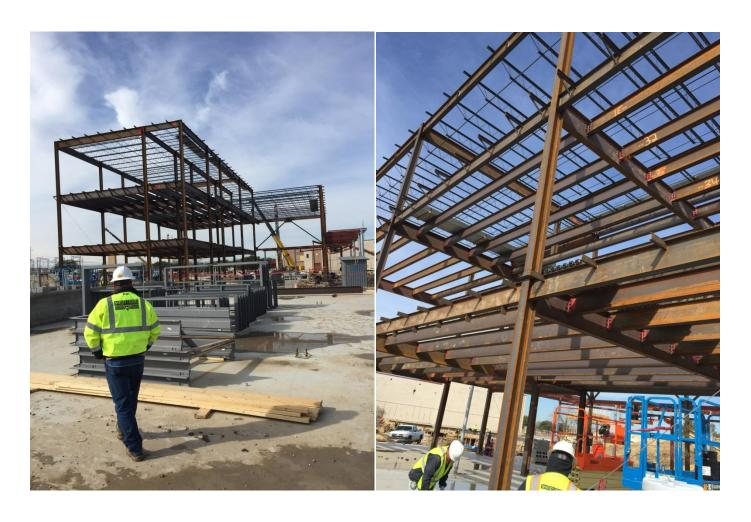
**STRUCTURAL** – Structural columns, beams and roof joists are being erected at the 3 story classroom area.
