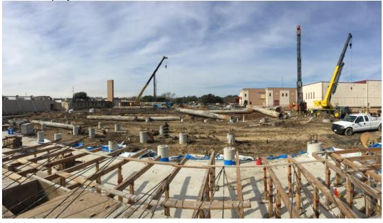
**PIERS** – Pier drilling continues just north of the current Cafeteria building. Steel casing (pipe) continues to be used as groundwater is encountered.
