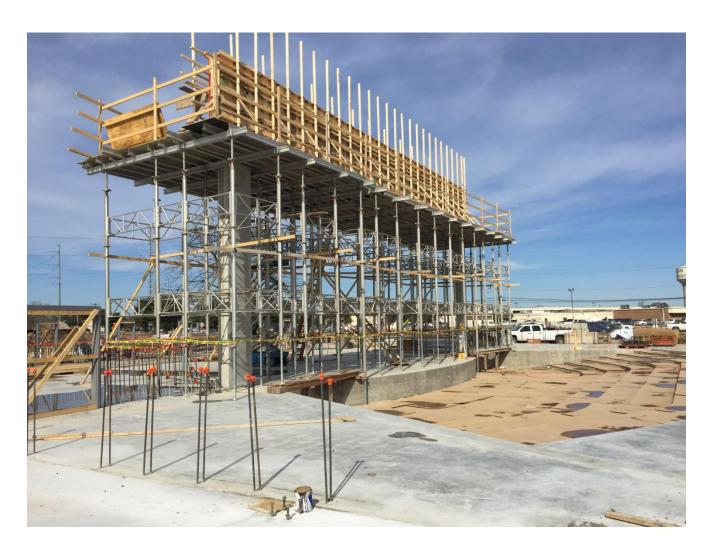
**CONCRETE STRUCTURE** – Formwork is being erected for the concrete beam that will span the Auditorium Stage opening.
